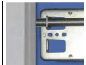
The deadbolt diameter is 5/8" A 3/4" hole, if drilled on center, should be sufficient. If you feel any rubbing, check to see which part of the bolt is rubbing on the hole and grind or enlarge that side of the hole.
